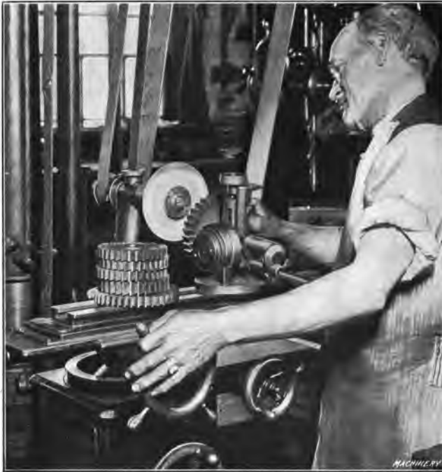
Fig. 12. Sharpening Side Milling Cutters
