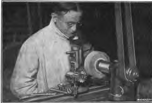
Fig. 20. Grinding the Clearance on End-mill Teeth
